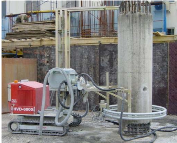
Typical Hydro-demolition Pile Breaker
