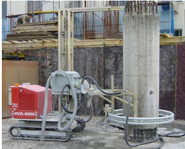
Typical Hydro-demolition Pile Breaker
