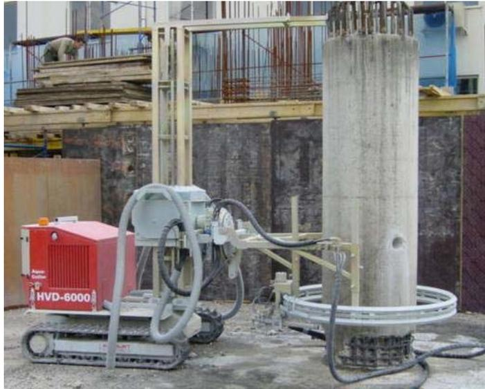
Typical Hydro-demolition Pile Breaker
