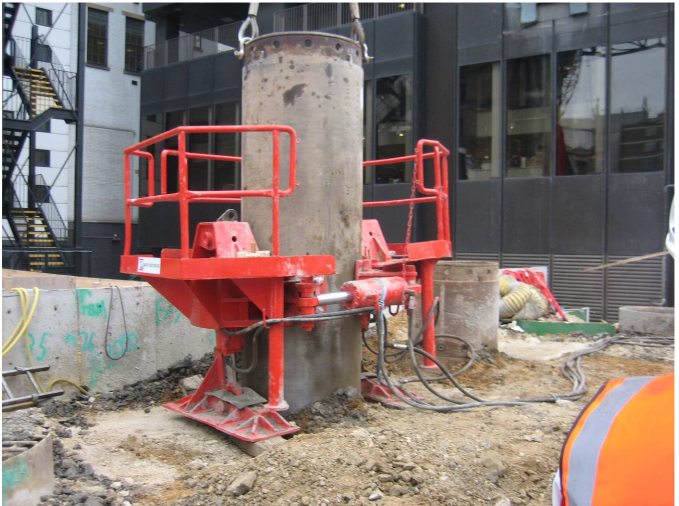
Figure 10. Purpose built casing extractor.
