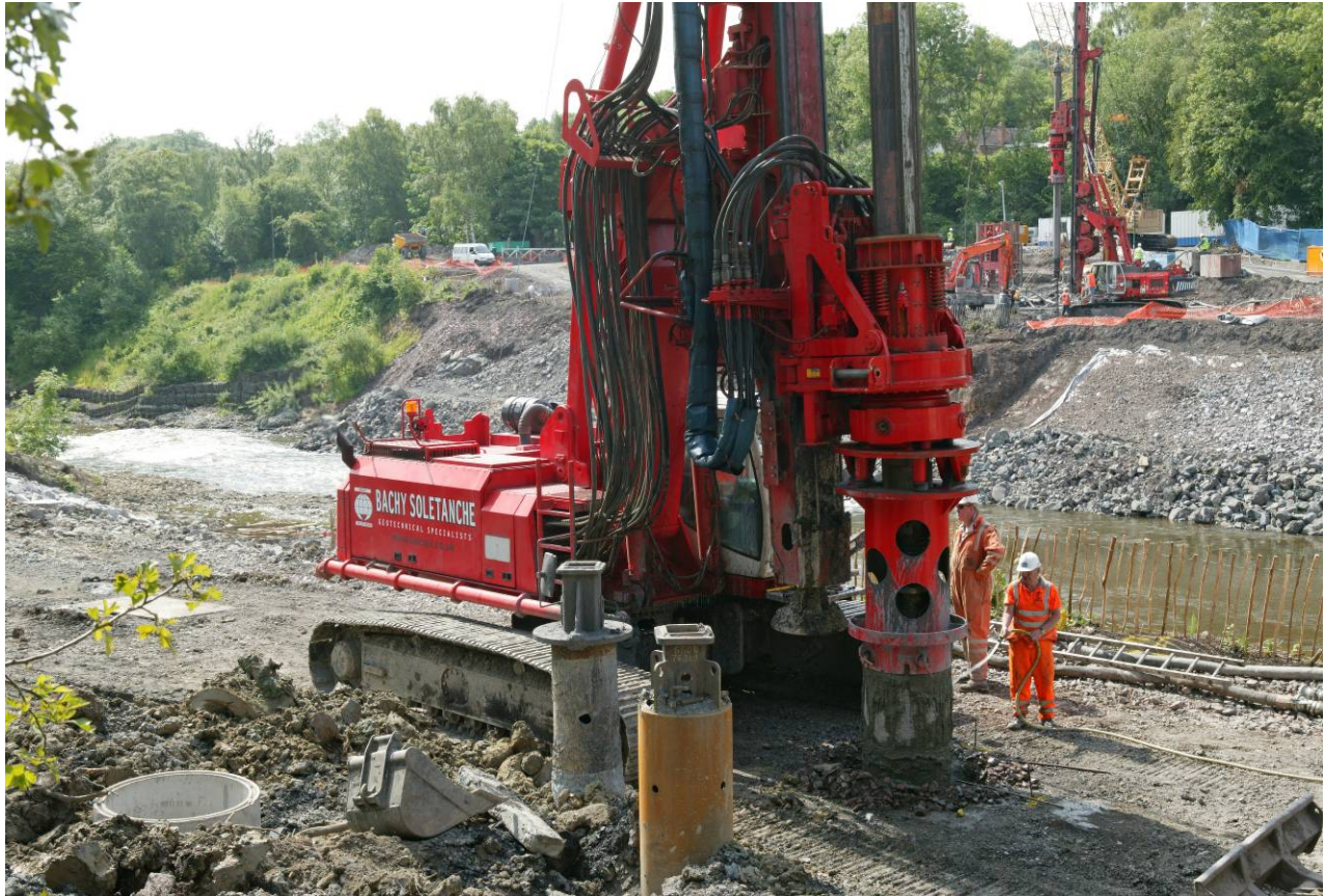
Figure 7. Hydraulic Piling rig with casing adaptor fitted to rotary table.
