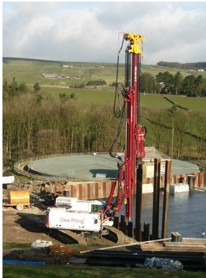
Figure 8. Hydraulic Piling Rig
