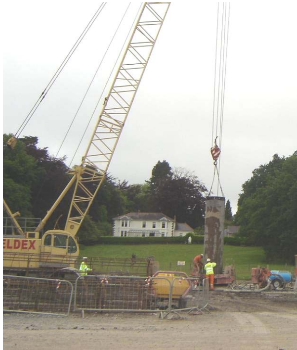
Figure 11. Crane extracting a length of segmental casing from a propriety oscillator
