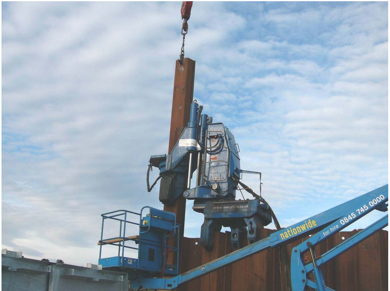
Figure 6. Propriety Jacking System in use with sheet piles.
