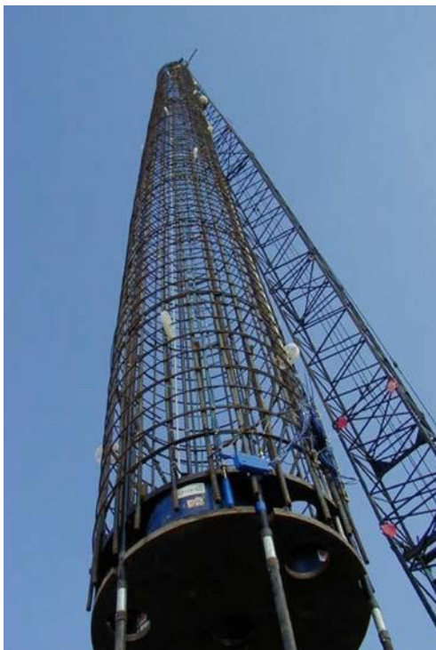
Figure 5.4 Load cell in reinforcement
