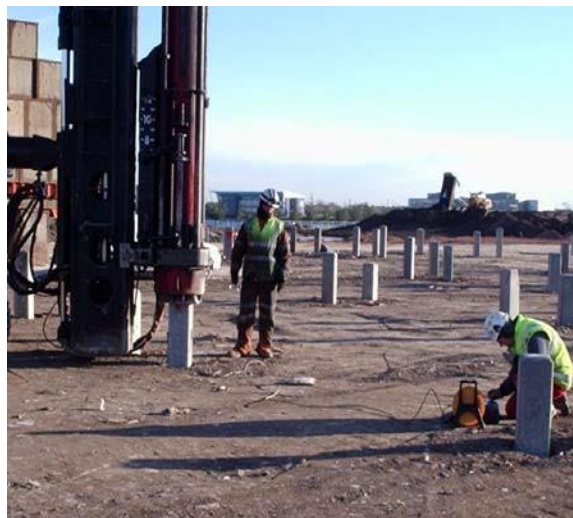
Figure 5.8 Dynamic load testing of driven precast concrete piles
