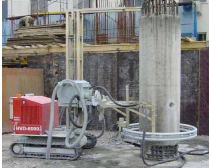
Typical Hydro-demolition Pile Breaker
