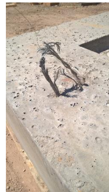
Example of damaged wire lifting loops
