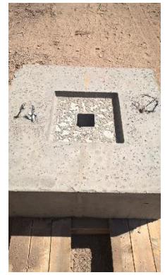
Example of damaged wire lifting loops
