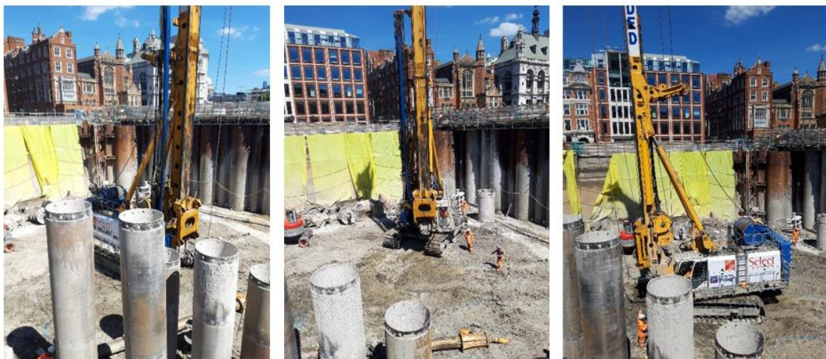
Rig starting position
