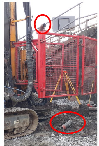
Swan neck arrangement of pipe that failed
